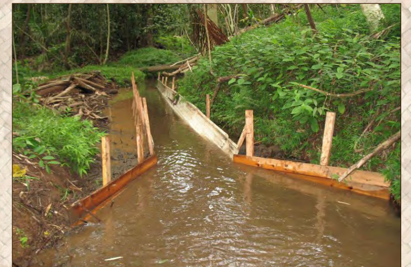
Temporary Repairs at Maunawili Ditch
